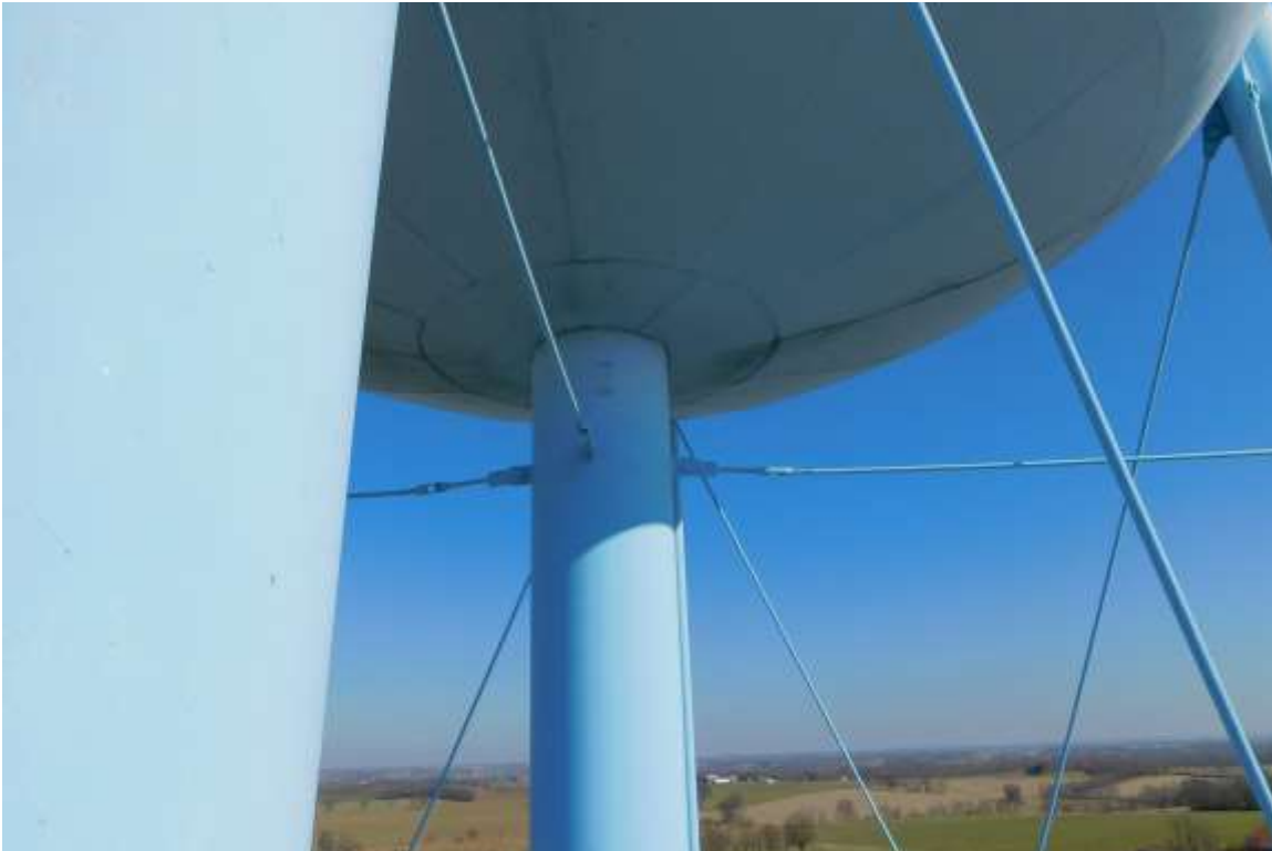
Photo shows the condition of the riser pipe and bowl. The connection appears to be in good condition.
